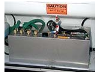
Illustration 1: The Hurricane Heater provides heat to the coach and on-demand domestic hot water.
